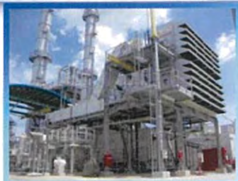
GTG : Elec.38 MW, Hot gas 562 °C X 6 Unit
